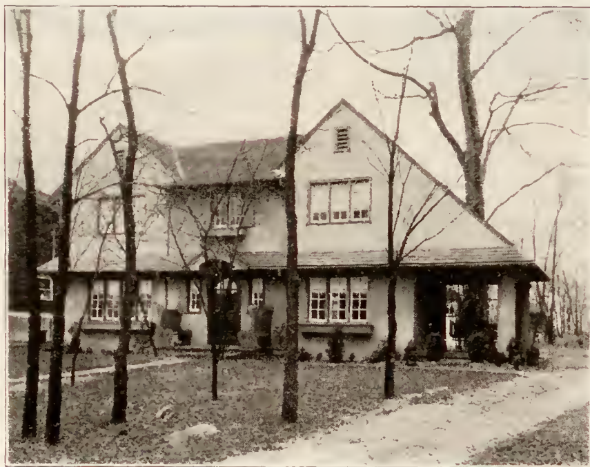
Typical Home near Chadwick Heights
